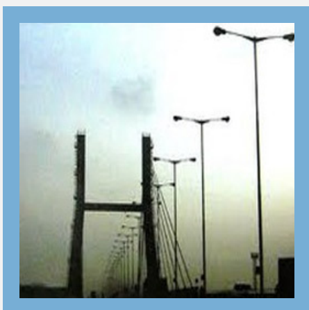
Street Light Poles
